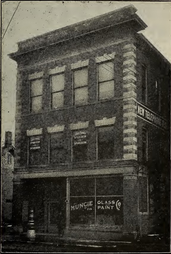
NEW D. & M. TELEPHONE BUILDING
