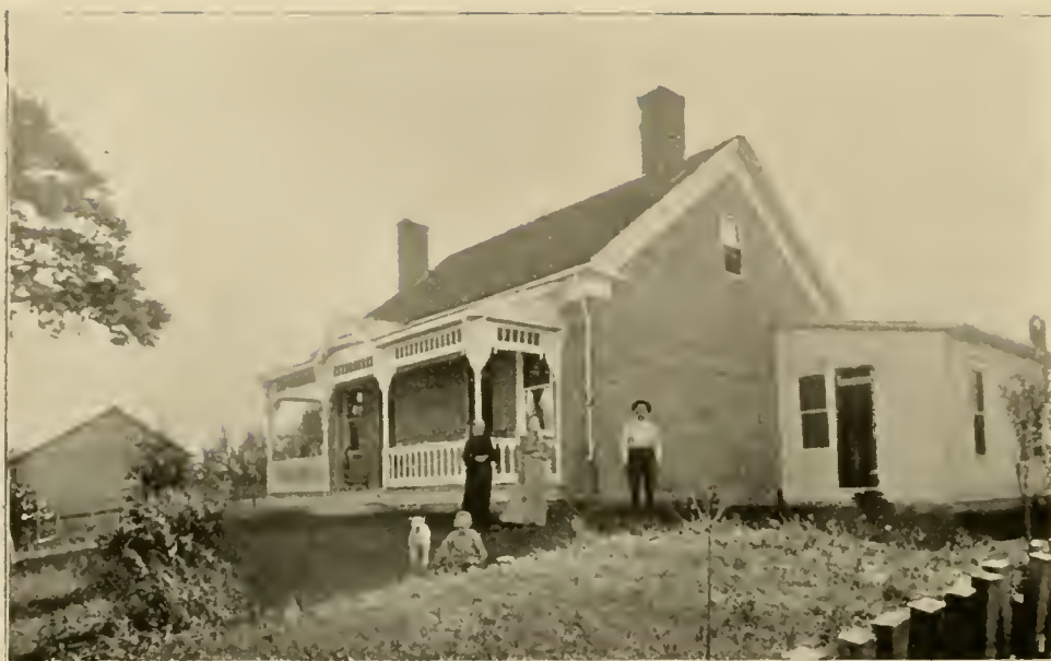
RESIDENCE AND FARM BUILDINGS OF ELISHA R. WINGATE, An old citizen and farmer of Delaware township, 7 miles northeast of Muncie. on the Granville pike.
